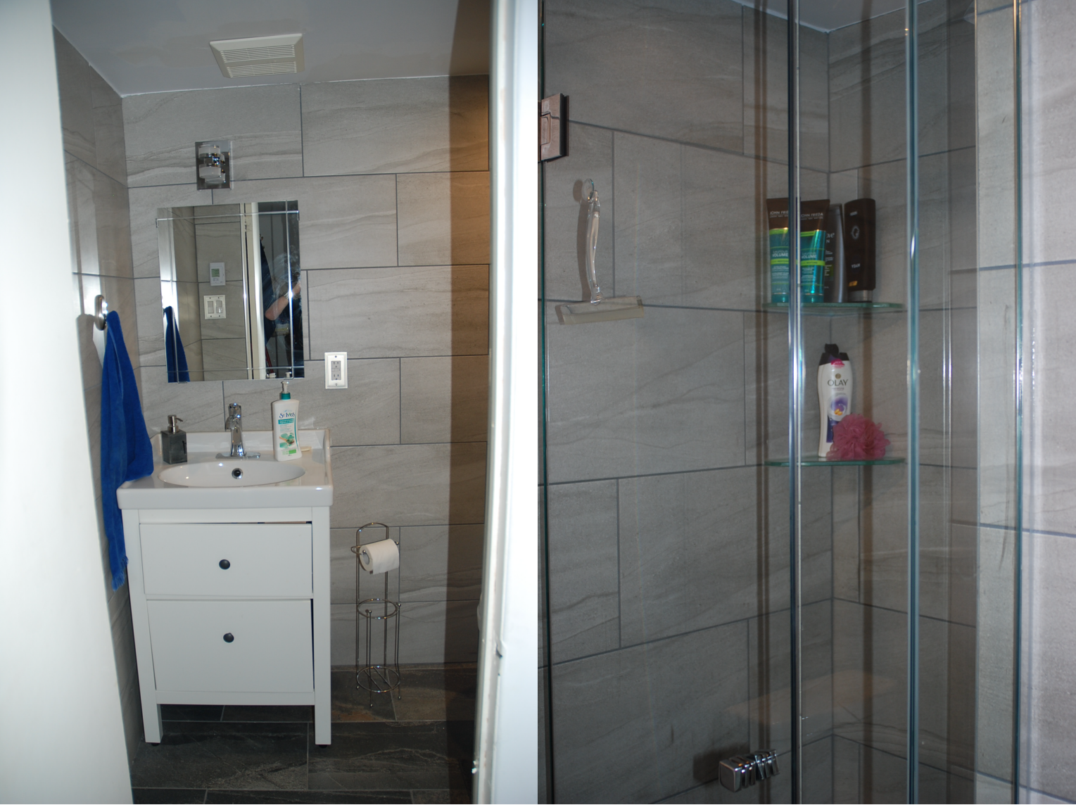
Bathroom renovation with Full wall tiles, heated tile floor
