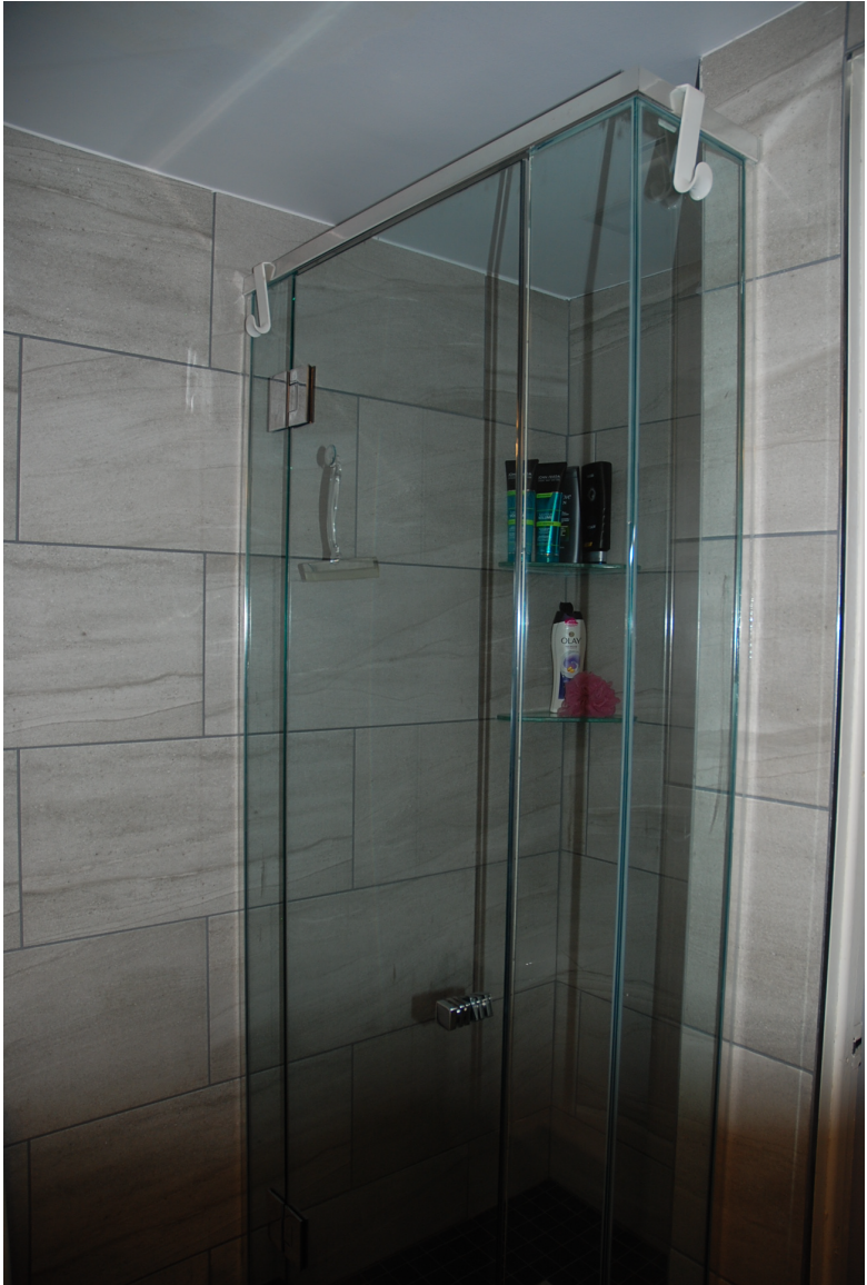
glass shower doors installed over custom size shower space
